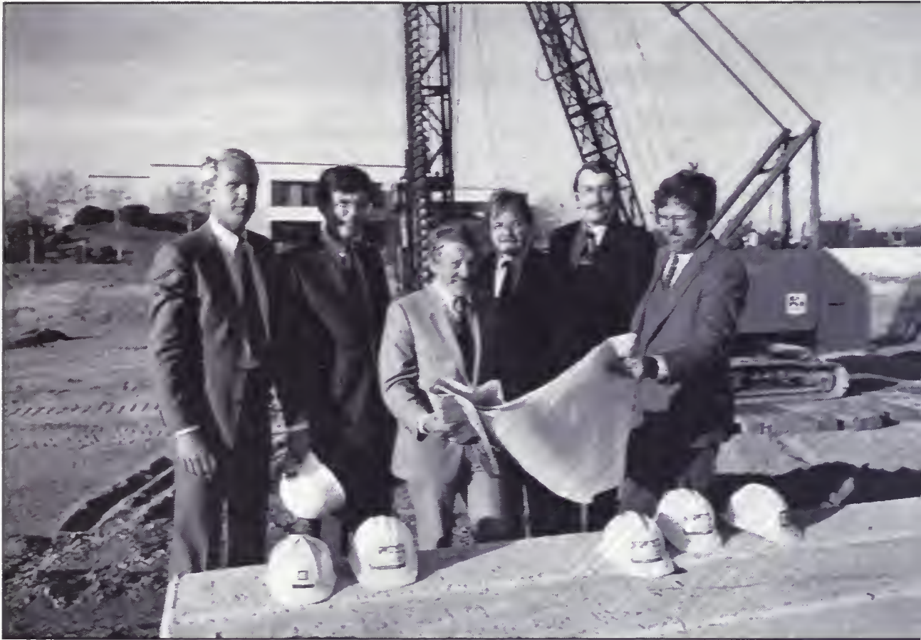
Fountain Valley Hospital groundbreaking, 1984. Left to right: Fountain Valley city official; Westcott Price, FHP; Robert Gumbiner, FHP; Harold Johnson, FHP; Randy Bosch, Project Architect; William Rosecrans, FHP.
